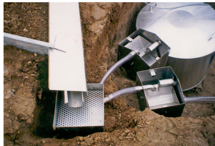
RUN-OFF MEASURING DEVICE - for recording and automated sampling of surface run-off. Inlet system, tilt counter, microcomputer-controlled autosampler.
